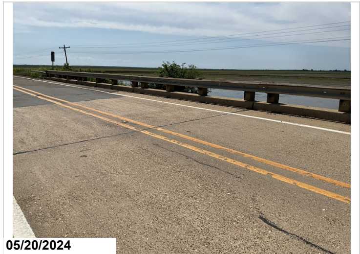
Span 14, Metal Bridge Railing, Right Side: 10' of minor collision damage. 10LF CS2 (Distortion)
