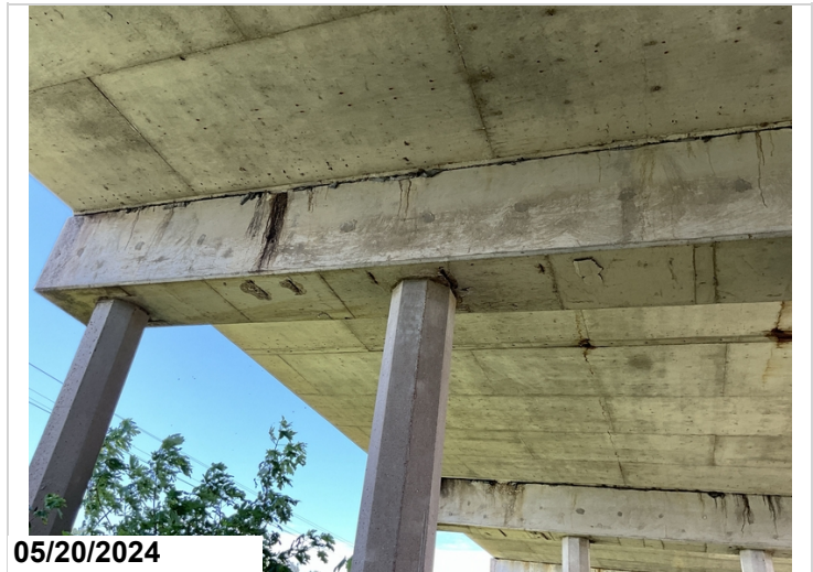
Bent 14, Pile Cap, Bottom: Five small pieces of exposed reinforcing steel. Reinforcing steel has minor section loss. 5LF CS3 (Exposed Rebar)
