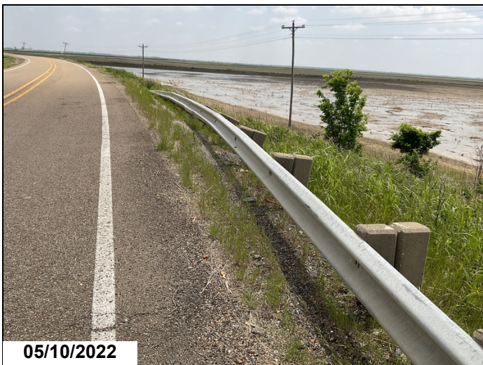
Abutment 2, Approach Rail, Right Side: Leaning out.
