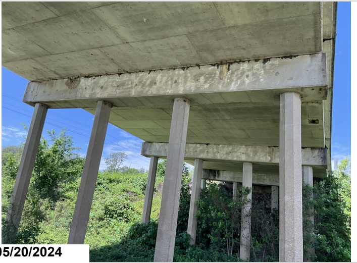
Bent 4, Pile Cap, Ahead, Top, Between Piles 3 & 4: 1' (Width) x 1 1/2' (Length) spall no exposed reinforcing steel. 2LF CS3 (Delamination/Spall/Patched Area)
