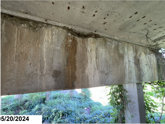
Bent 16, Pile Cap, Ahead, Left End, Between Piles 1 & 2: Three 1' (Length) x 6" (Height) spalls no exposed reinforcing steel. 3LF CS3 (Delamination/Spall/Patched Area)
