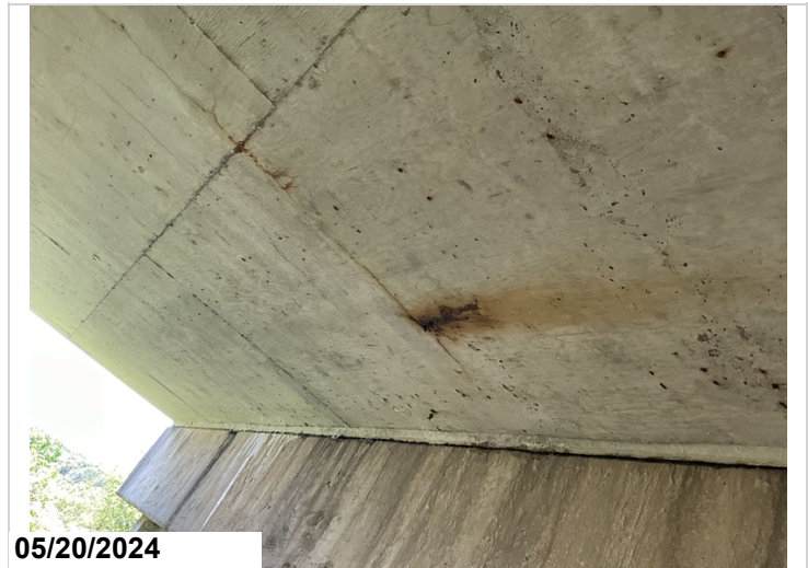
All Spans, Deck Undersurface, Full Length: Hairline cracks with rust staining. 400SF CS3 (Efflorescence/Rust Staining)
