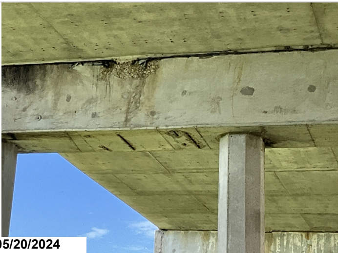
Bent 13, Pile Cap, Ahead, Top, Between Piles 3 & 4: 1' (Width) x 1 1/2' (Length) spall no exposed reinforcing steel. 2LF CS3 (Delamination/Spall/Patched Area) Bent 13, Pile Cap, Bottom, Right: Six small pieces of exposed reinforcing steel. Reinforcing steel has minor section loss. 2LF CS3 (Exposed Rebar)
