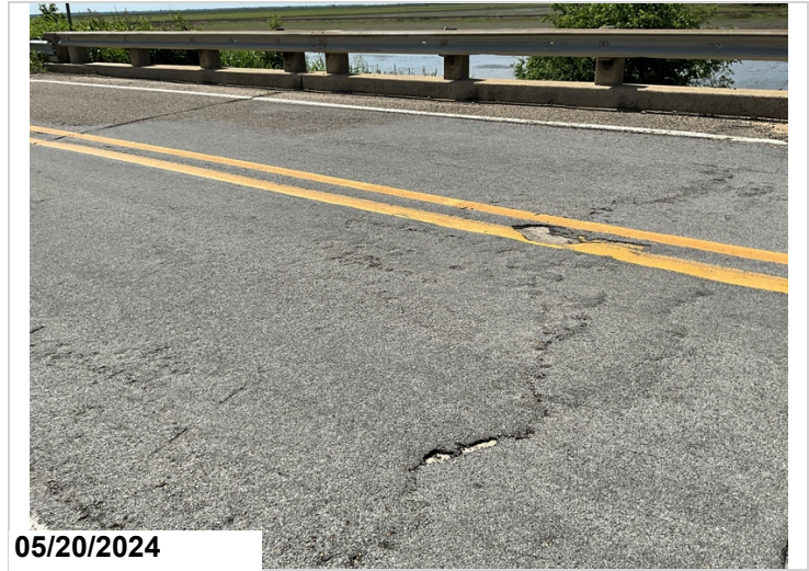
Span 15, Wearing Surface: Two small shallow spalls. 2SF CS2(Delam/Spall/Patched Area/Pothole)
