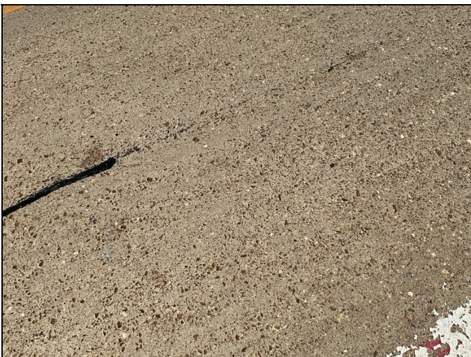
All Spans, Deck Surface: Transverse and longitudinal cracks. 1800SF CS2 (Cracking)
