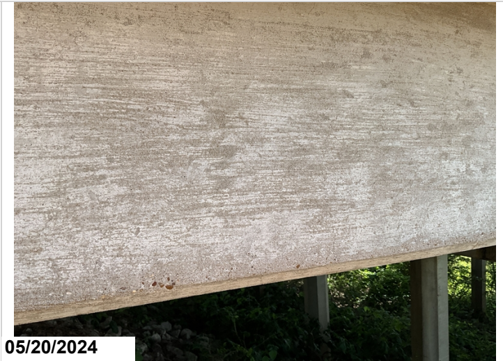
All Spans, Slab, Both Sides: Vertical hairline cracks.
