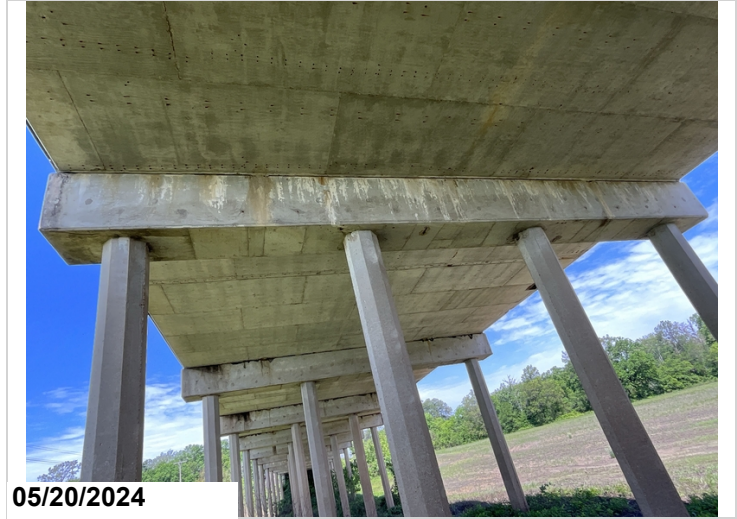
Bent 12, Pile Cap, Bottom: Three small pieces of exposed reinforcing steel. Reinforcing steel has minor section loss. 3LF CS3 (Exposed Rebar)
