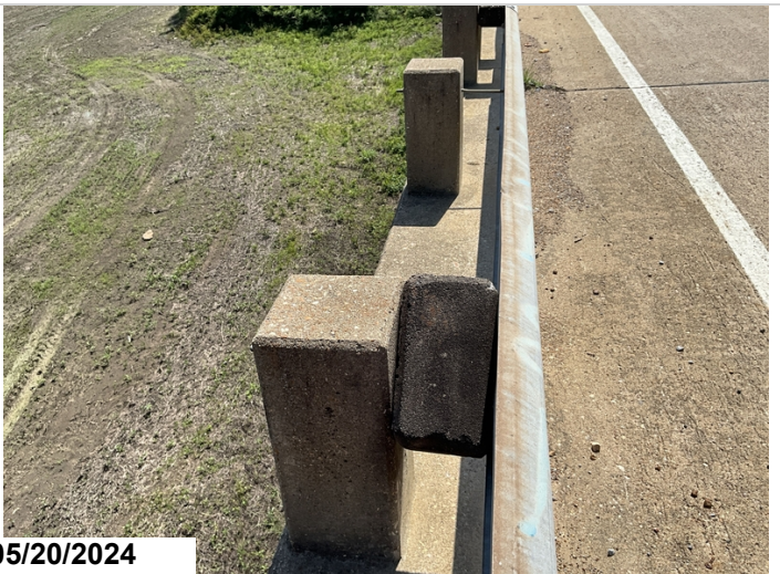
Span 9, Metal Bridge Railing, Left Side: One missing rail post spacer. 1LF CS3 (Connection)
