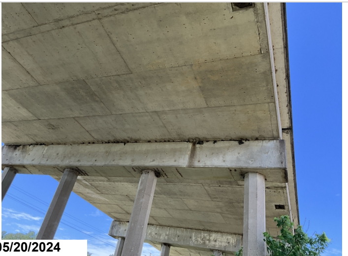
Bent 7, Pile Cap, Bottom, Full Length: Twelve small pieces of exposed reinforcing steel. Reinforcing steel has minor section loss. 9LF CS3 (Exposed Rebar)
