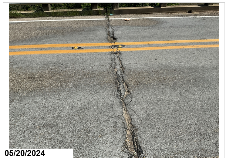
Span 1, Wearing Surface, Bent 2 Joint: Shallow spalls in left lane. 28SF CS2 (Delam/Spall/Patched Area/Pothole)
