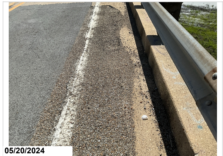
All Spans, Gutters, Full Length: Dirt and debris.
