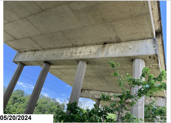
Bent 6, Pile Cap, Bottom, Left End: Two small pieces of exposed reinforcing steel. Reinforcing steel has minor section loss. 1LF CS3 (Exposed Rebar)
