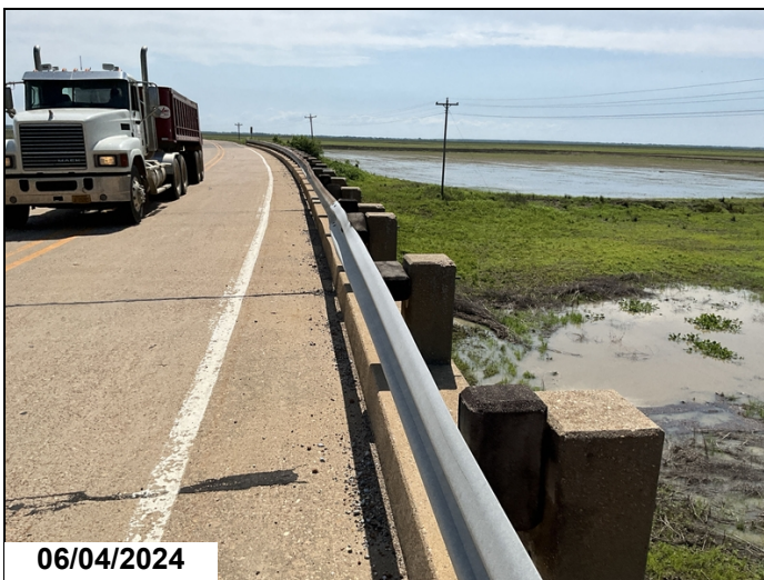
Span 4, 5 & 6, Metal Bridge Railing, Right Side: 30' of minor collision damage. 30LF CS2 (Distortion)
