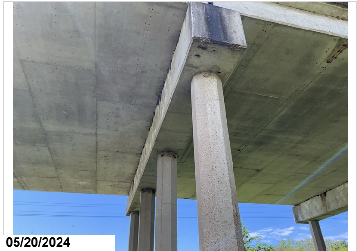
Bent 4, Pile Cap, Bottom, Left End: Three small pieces of exposed reinforcing steel. Reinforcing steel has minor section loss. 2LF CS3 (Exposed Rebar)
