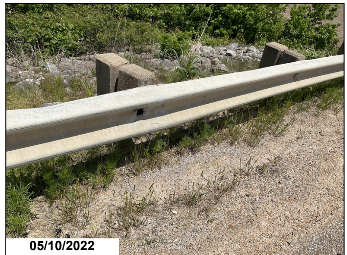
Abutment 1, Approach Rail, Left Side: Seventh post is not connected.
