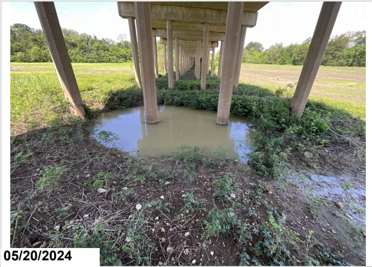
Bent 13 area of minor scour
