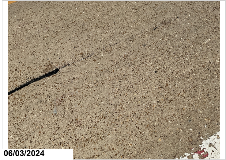
All Spans, Deck Surface: Transverse and longitudinal cracks. 1800SF CS2 (Cracking)
