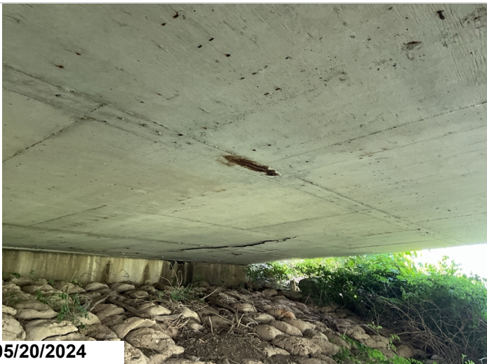
Span 16, Deck Undersurface, Right, Near Abutment 2: 4' (Length) X 2' (Width) delaminated area. 8SF CS2 (Delamination/Spall/Patched Area)
