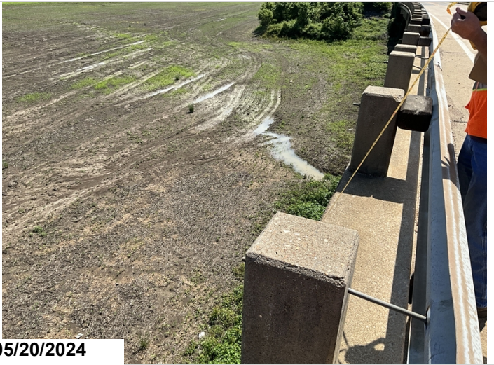
Span 6, Metal Bridge Railing, Left Side: Two missing rail post spacers. 2LF CS3 (Connection)
