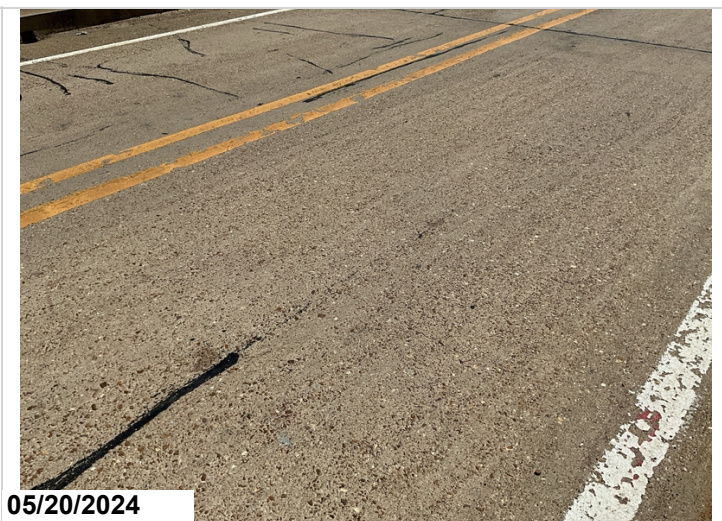
All Spans, Deck Surface, Full Length: Light abrasion. 4000SF CS2 (Abrasion/Wear)
