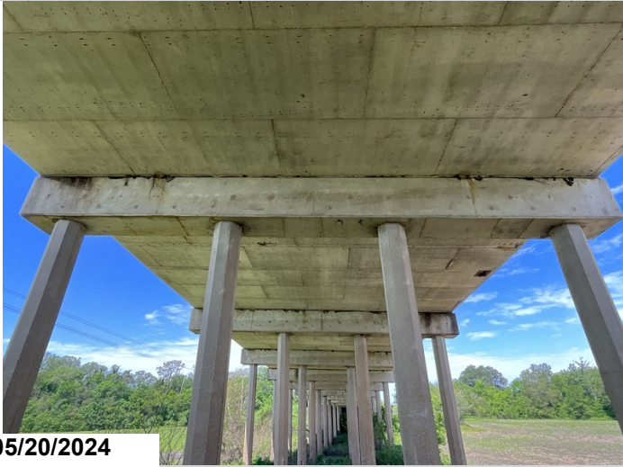
Bent 11, Pile Cap, Bottom, Near Center: Two small pieces of exposed reinforcing steel. Reinforcing steel has minor section loss. 2LF CS3 (Exposed Rebar)
