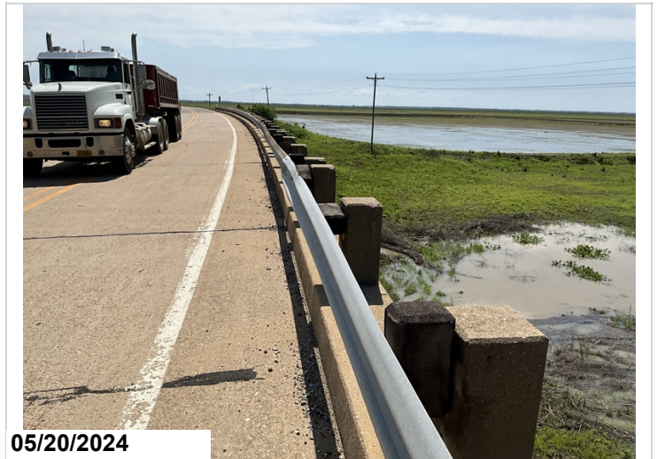
Span 4, 5 & 6, Metal Bridge Railing, Right Side: 30' of minor collision damage. 30LF CS2 (Distortion)
