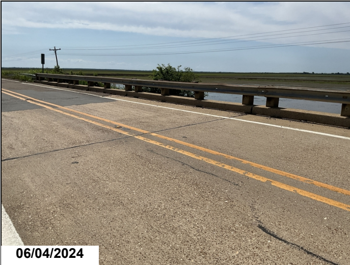
Span 14, Metal Bridge Railing, Right Side: 10' of minor collision damage. 10LF CS2 (Distortion)
