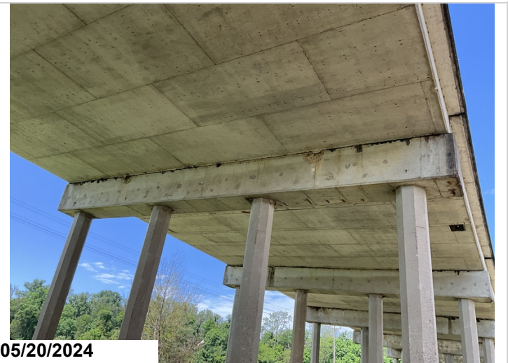
Bent 9, Pile Cap, Ahead, Top, At Keyways: 1' (Width) x 1 1/2' (Length) spalls no exposed reinforcing steel. 4LF CS3 (Delamination/Spall/Patched Area) Bent 9, Pile Cap, Bottom, Left Half: Nine small pieces of exposed reinforcing steel. Reinforcing steel has minor section loss. 5LF CS3 (Exposed Rebar)
