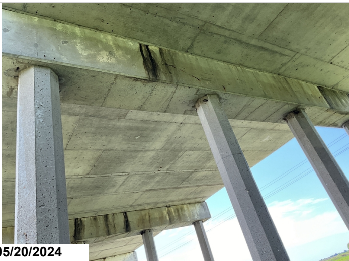
Bent 4, Pile Cap, Back, Near Center: 2; (length) cage steel exposed. Cage steel has minor section loss. 2LF CS3 (Exposed Rebar)
