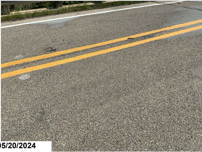
Span 1, Wearing Surface: Two small shallow spalls. 2SF CS2 (Delam/Spall/Patched Area/Pothole)
