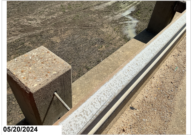
Span 7, Metal Bridge Railing, Left Side: One missing rail post spacer. 1LF CS3 (Connection)
