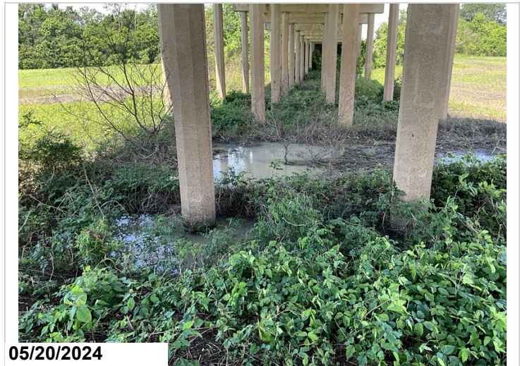
Typical scour around interior bents.
